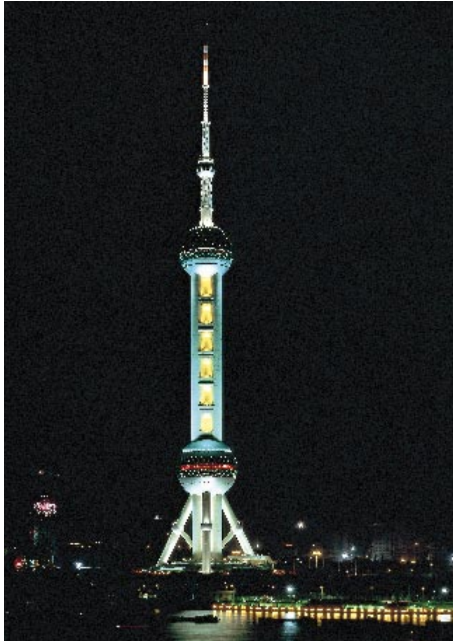
An Electrosonic Imagine system controls the exterior lighting of the Shanghai TV Tower – the tallest tower in Asia.
