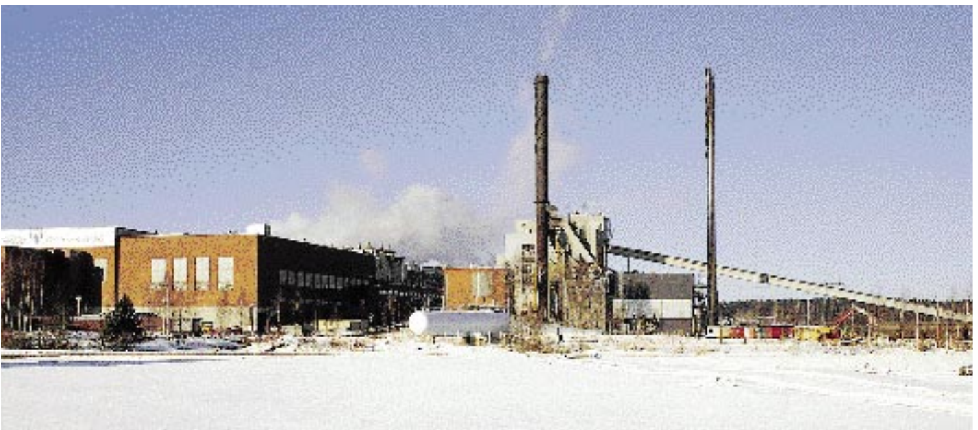
The Kirkniemi turnkey contract comprises a new natural-gas-fired power plant, the combining of the old and the new power plant, and a boiler to generate steam.
