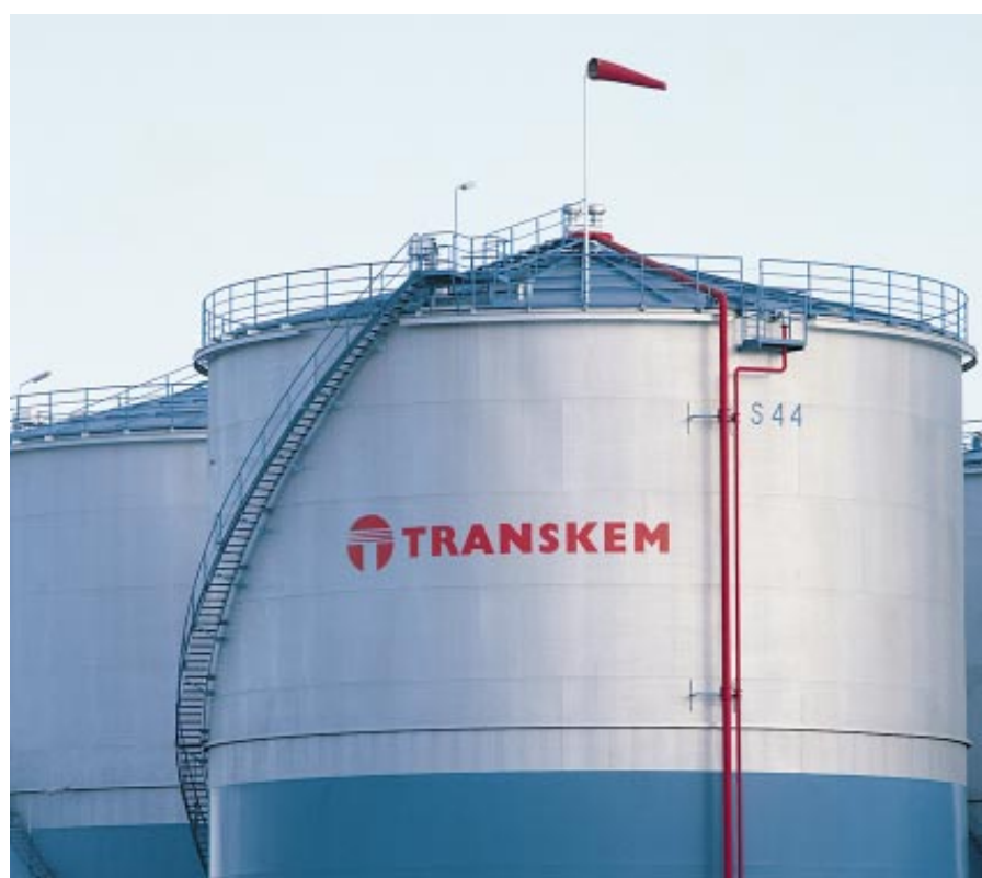
The top-flight tank terminal at Mussalo in Kotka serves the transit cargoes of liquid chemicals.
