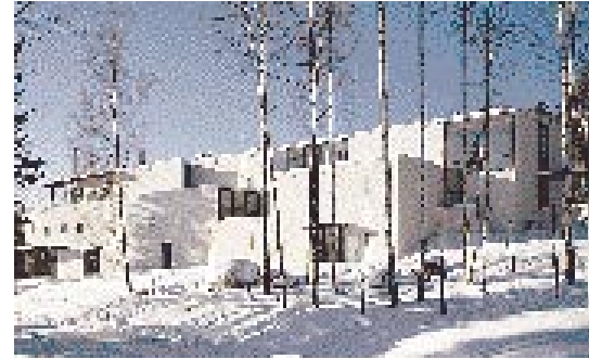
The laboratory of the Geodetic Institute in Kirkkonummi makes measurements which do not tolerate any vibrations. The state-of-the-art architecture building is anchored in solid Finnish bedrock.
