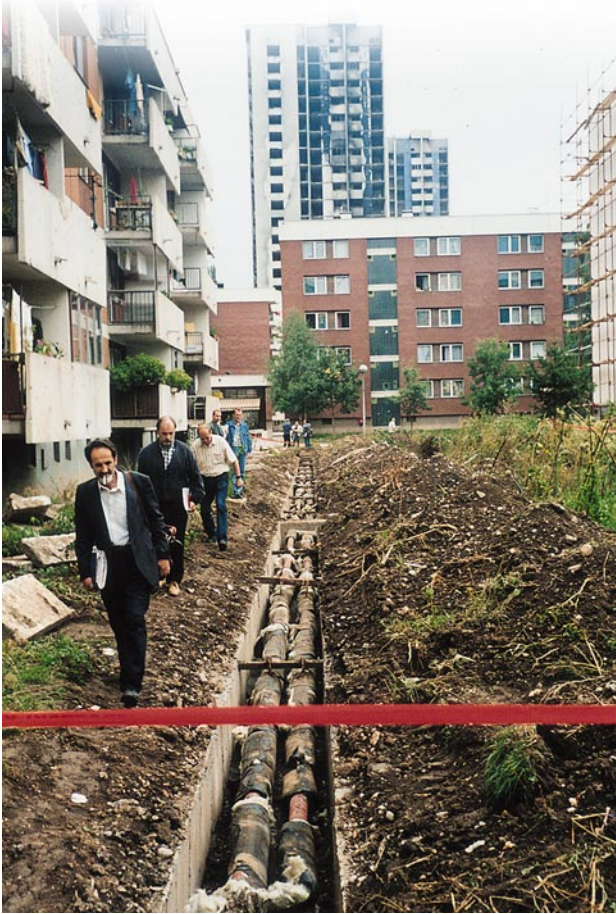
During the summer, more than 30,000 households in Sarajevo were connected to district heating using ABB Ecopipe's elements.
