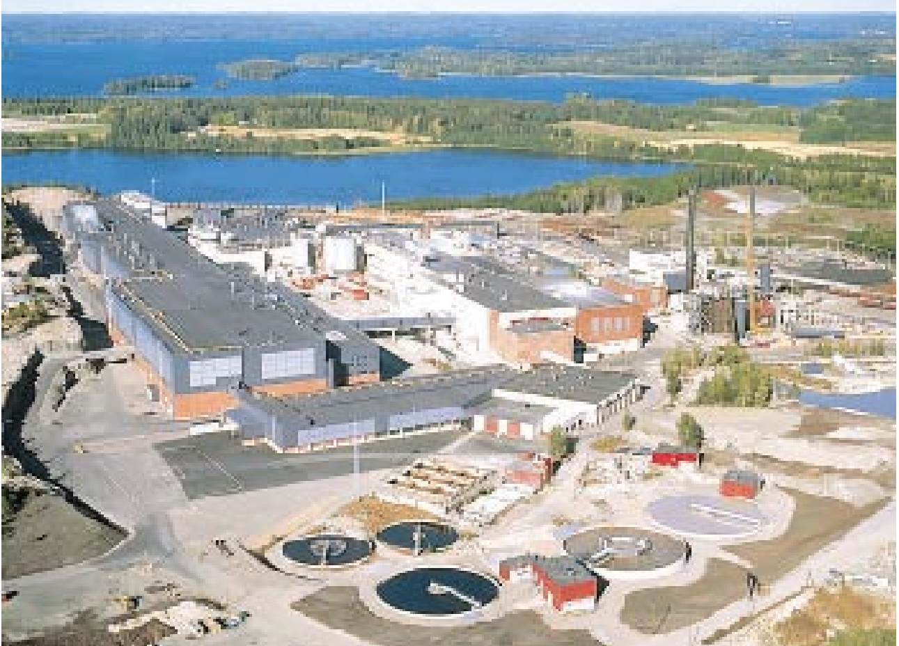
The new fine paper production line at Metsä-Serla's Kirkiniemi mill in Finland was started up in August 1996, well ahead of schedule. Jaakko Pöyry Oy was the main engineering consultant in this FIM 2.4 billion investment project.
