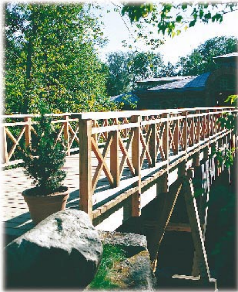
The bridge leading to the Granary at Fiskars village was built of local larch.
