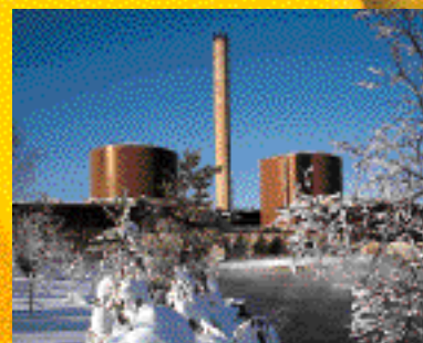
An extensive modernisation and power uprating project is being implemented at the Loviisa power plant.
