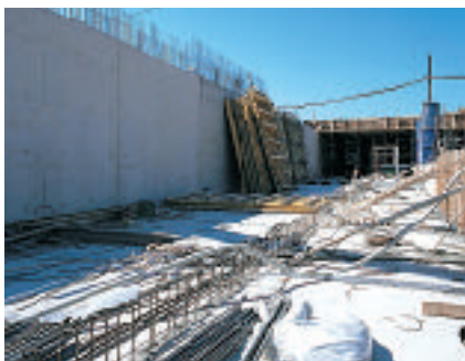
Commuter railway site at Puotila in Helsinki.
