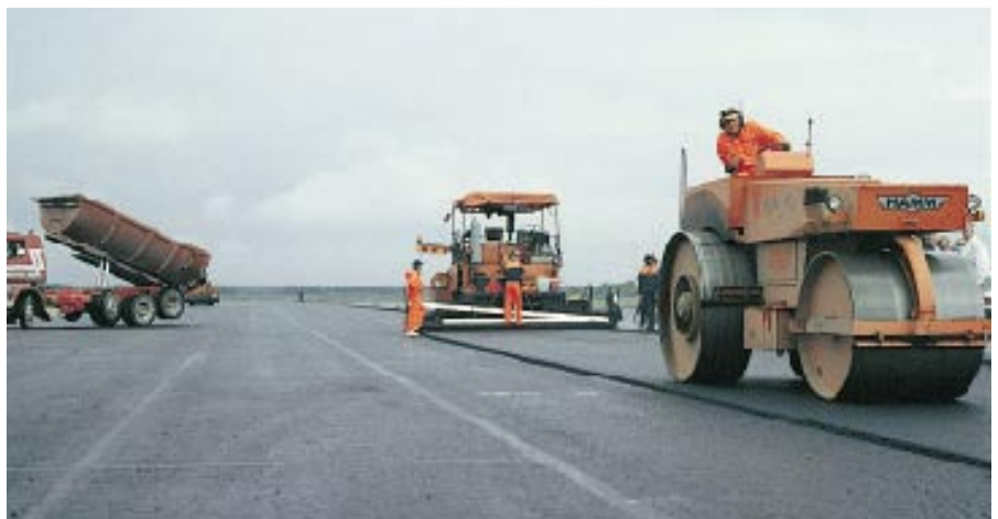
Pavement re-surfacing at Kauhava airport.
