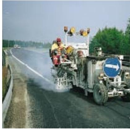
Spray applied road marking.
