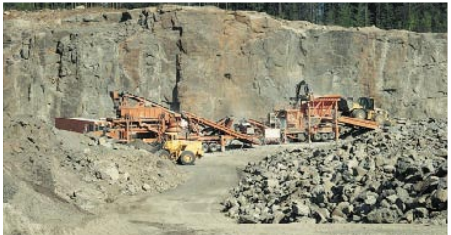
A transportable crushing plant.
