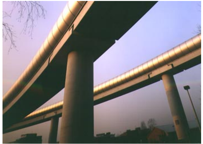
The Dutch company Spanbeton was awarded by the International Bureau for Precast Concrete for its outstanding precast concrete project: the curved bridge deck of the Amsterdam subway. Spanbeton is delivering similar bridge elements for a ring road project in Rotterdam.
