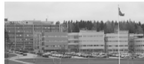
Polar built new offices and research facilities for Oy LM Ericsson Ab in Kirkkonummi.
