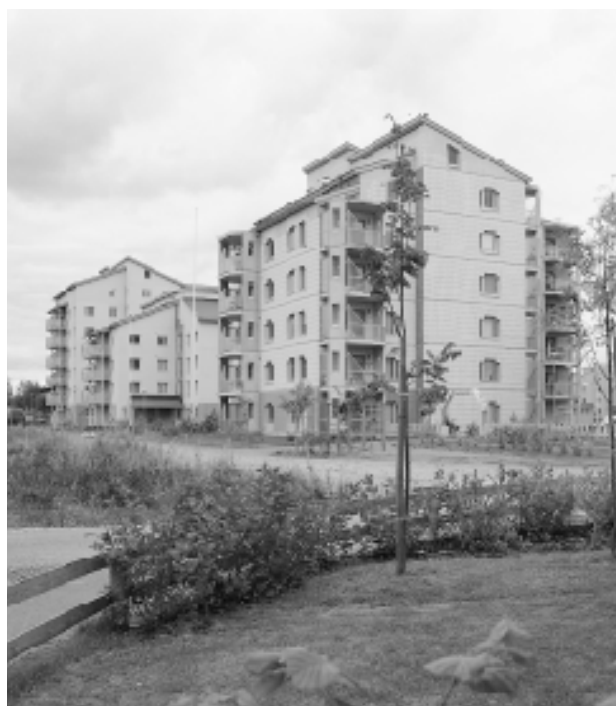
The Sandbacka residential area of Pakkala-Tammisto district in Vantaa is the first to be under construction. Four hundred dwellings have been completed. Some 1,000 people live in Sandbacka.
