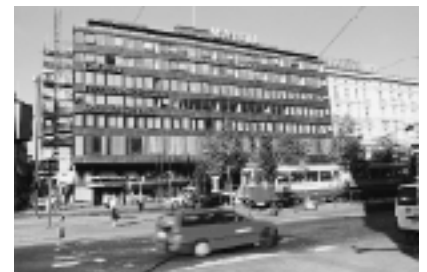
Polar renovated the prestigious Hotel Marski, owned by Arctia Oy, which went into business in the early 1960s.
