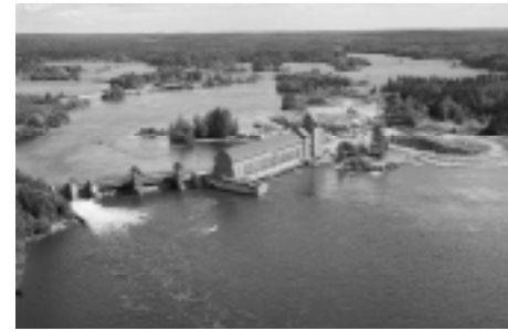
The Äetsä power plant was completed in 1996. Polar's Eastern Finland unit performed the construction engineering work for the new machinery station of UPM-Kymmene Corporation's Äetsä power plant.
