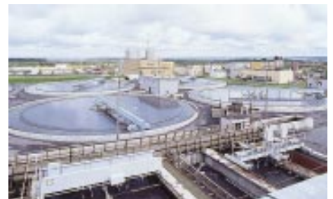
Uppermost picture: Waste water clarification basins under construction for the Joutseno Pulp Mills of UPM-Kymmene Oy, Joutseno.
