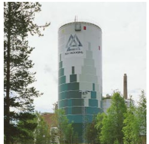
Prefabrication of high pressure piping at the Ylivieska factory of YIT Power Oy. A pulp storage tower, including installation, delivered to SCA, Piteå, Sweden.
