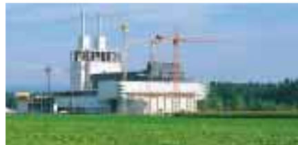
Thermal waste treatment plant Thurgau in Switzerland
