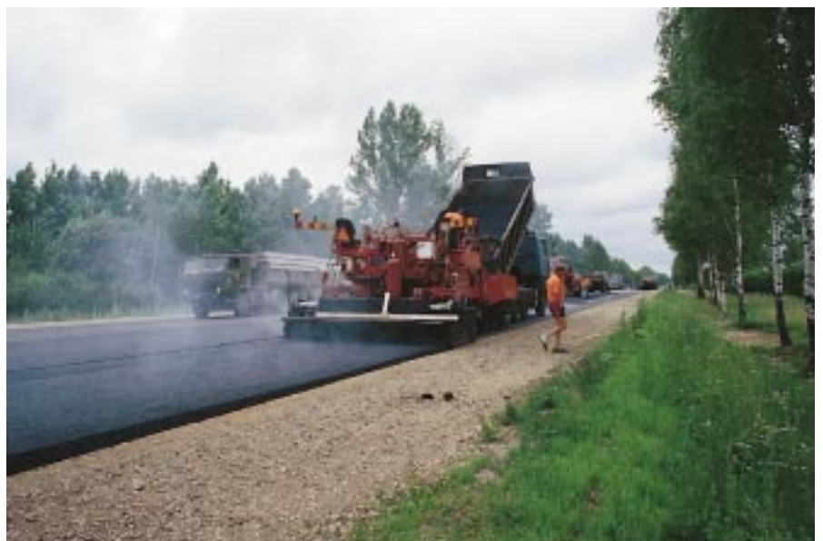
Paving work in progress on the Moscow-Minsk highway.
