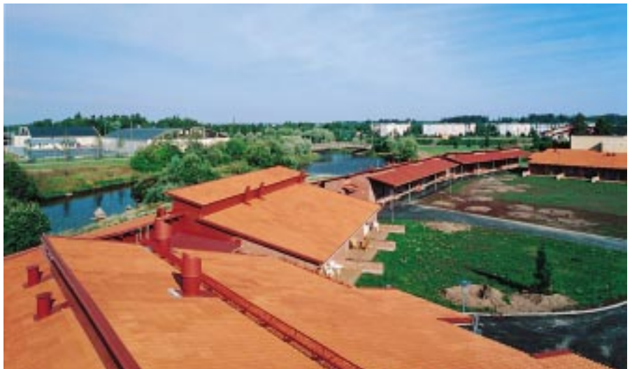
Huittinen old persons' service centre with its new tiled roof.
