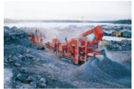
Stone crushing plant at Suomenoja in Espoo.
