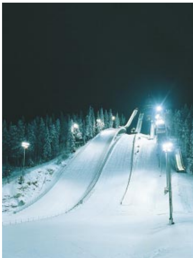
Savocon Oy constructed the K 120 ski-jumping hill at Puijo, Kuopio.
