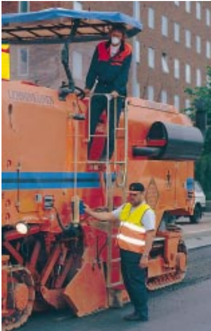
Milling plant and crew at work.
