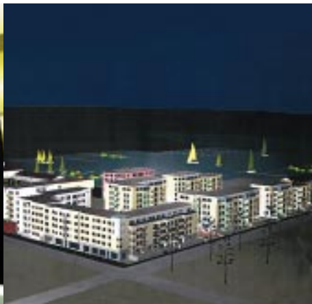
Privately financed dwellings are under construction at Kuopio harbour. A home of your own in the centre of town and beside a lake – the Finnish dream.
