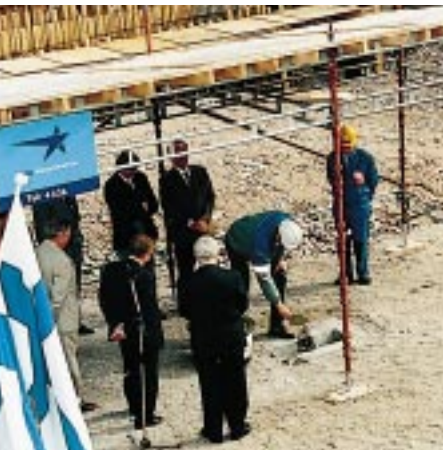
Laying the foundation stone at Pitkälkoski. The active carbon filtering plant purifies the water piped in to potable quality close to aquifer standards.
