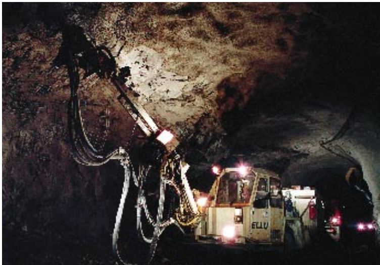
The new user-friendly concrete spraying machine delivered by Normet is reinforcing the walls of an underground tunnel in the Pyhäsalmi mine of Outokumpu Mining Oy, Finland.
