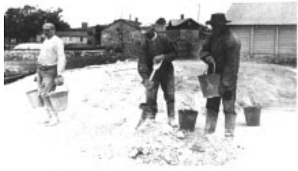
Quick lime was slaked initially by hand using sea water. Pargas c. 1910.
