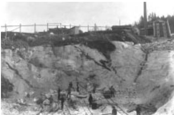
Crushed limestone was transported in rail carts. Limberg quarry, Pargas c. 1910.
