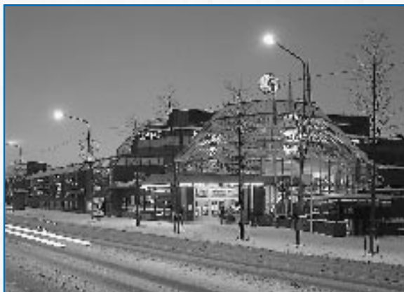
The Koskikeskus complex in the heart of Tampere is Polar's biggest shopping centre. Ten years old, this varied complex has a 100% rental occupancy rate.
