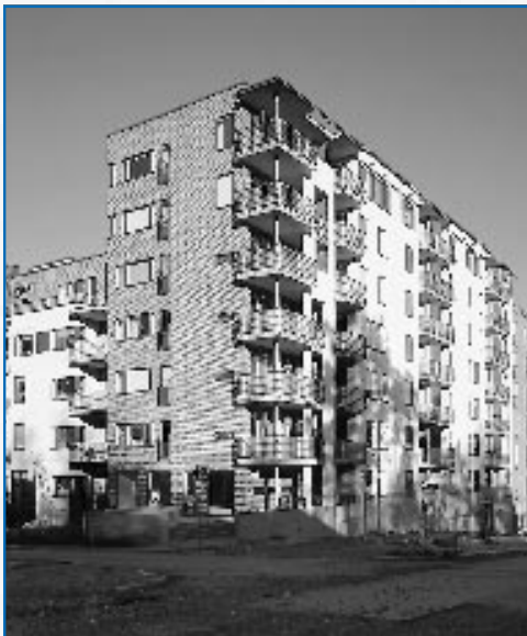
Tenant-owner homes on Takomatie in the Pitäjänmäki district of Helsinki, built for the VVO Group.
