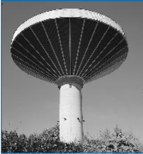
The mushroom model is a popular solution for many of the water towers built by Polar under contract throughout the land. The picture shows the Kuokkala water tower built for the Jyväskylä Water Utility.
