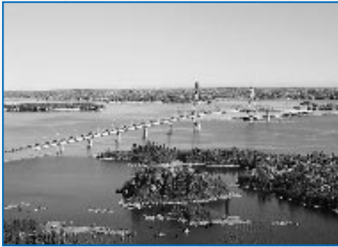
Finland's longest bridge, at Raippaluoto near Vaasa, was opened to traffic two months ahead of schedule in August 1997. The client was Vaasa Regional Road Administration.
