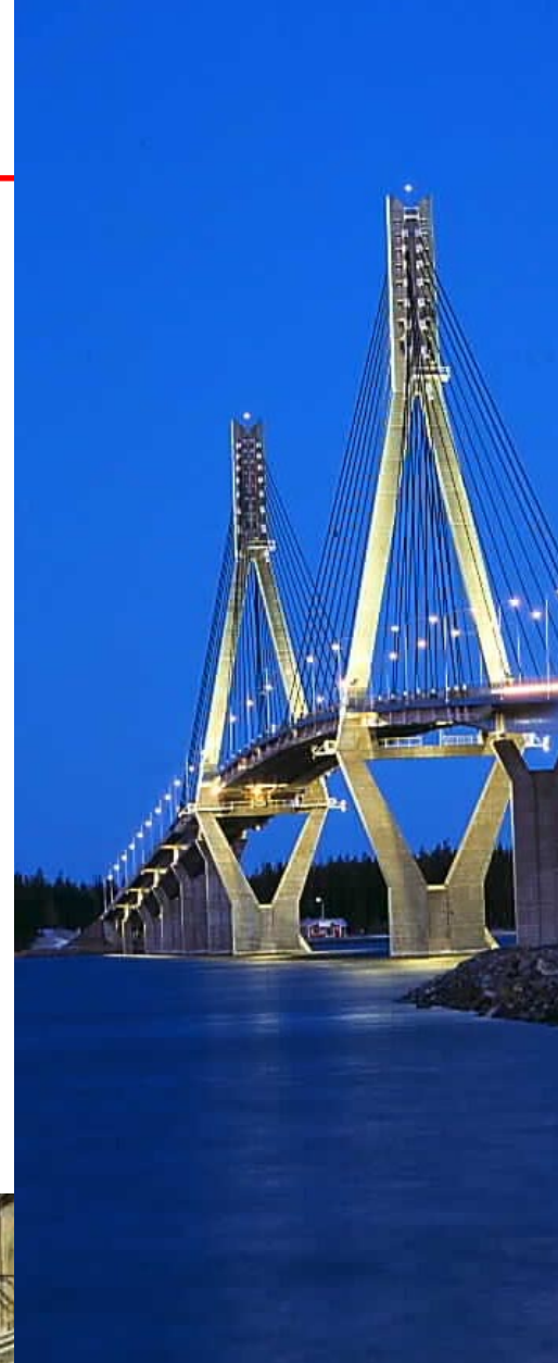
Finland's longest bridge Raippaluoto Bridge was completed last autumn. More than 3000 tonnes of Rautaruukki's fine-grained structural steel was used in its structures.
