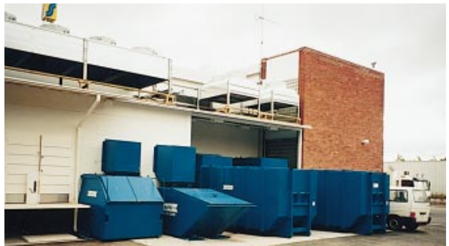
Waste produced by the Konala S Market is sorted into four containers: mixed waste (left), organic waste, energy waste and cardboard.
