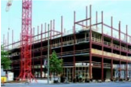
Among the advantages of a steel frame are its fast installation time. The steel frame of the Kiinteistö Oy Itämerenkatu 3 office and commercial building in Helsinki's Ruoholahti district.
