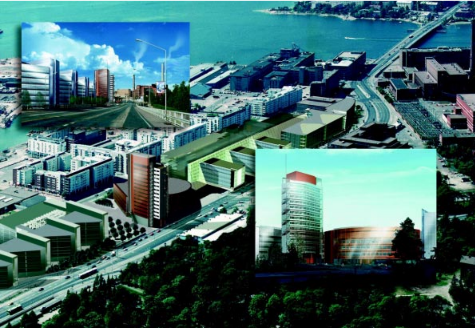
The 16-storey Kiinteistö Oy Itämerentori office building is being erected within the Ruoholahti shopping and office building complex and will become the western landmark of the Helsinki cityscape. YIT has a number of major construction projects either under way in the area or in the pipeline.
