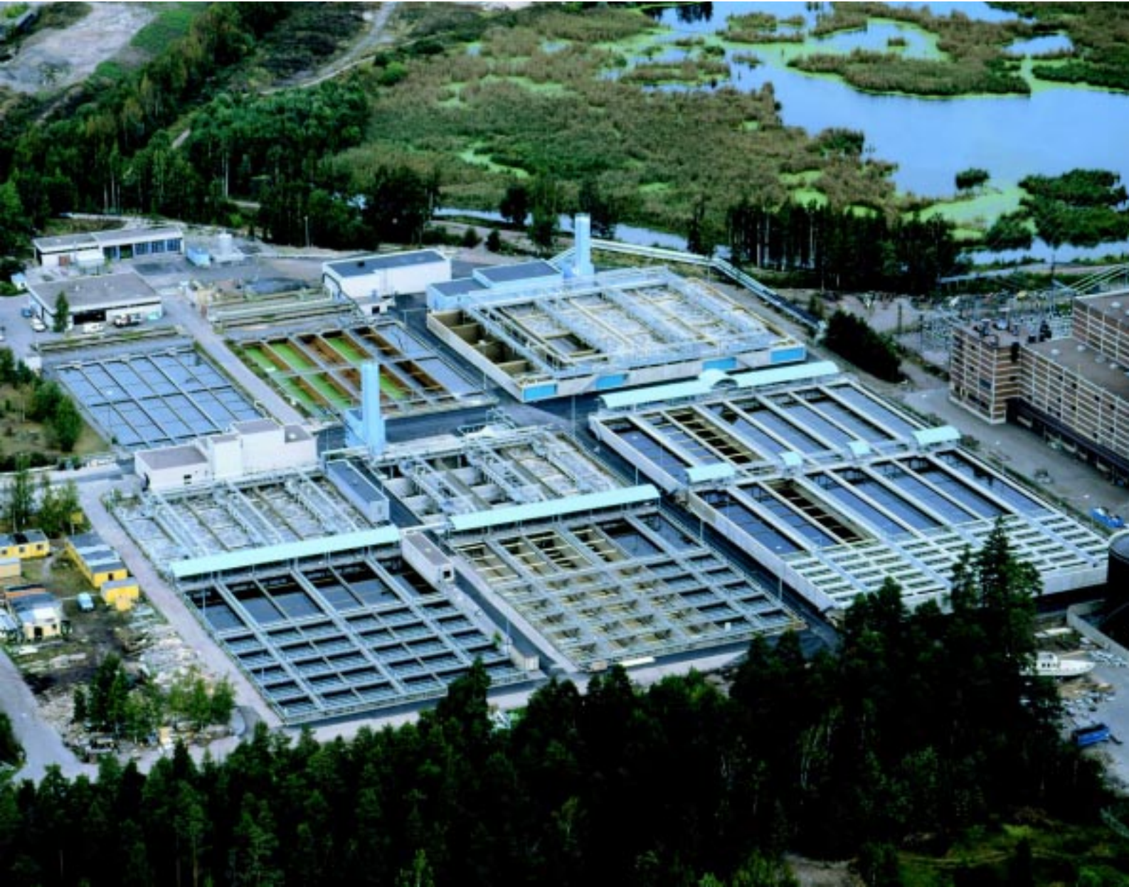
The denitrification unit of the Suomenoja waste water treatment plant is the first of its kind in Finland. The total volume of the new pools and buildings is 73,000 cu.m.
