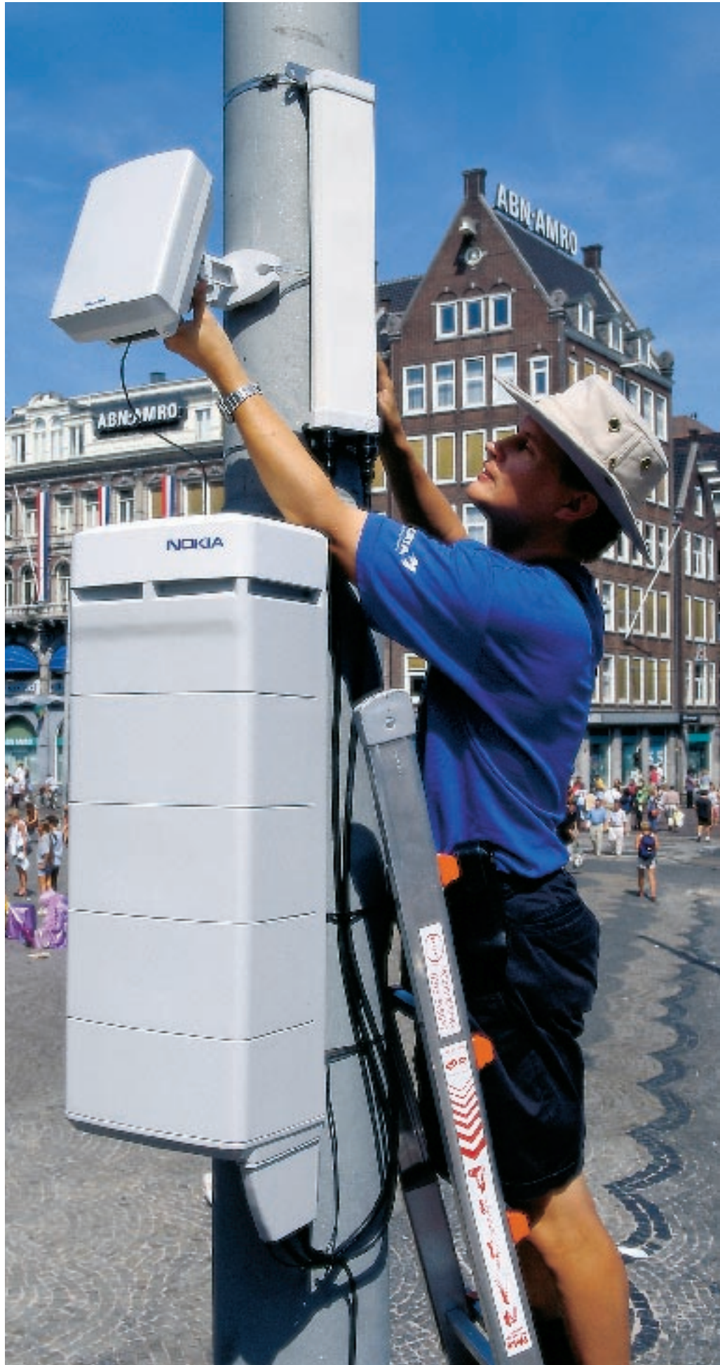
New Nokia MetroSite Base Station. Telecommunications applications comprise close to 80% of all Efore products.
