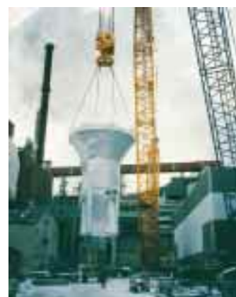
Lifting the reactor, Husum tall oil plant, Sweden
