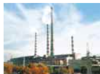
Bishkek district heating power plant, Kirgisia
