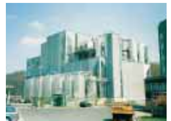
Xylose production plant, Austria
