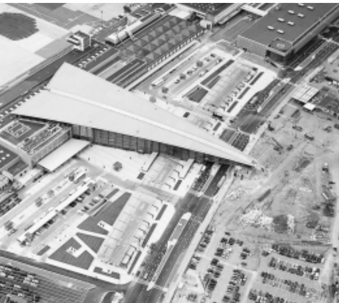
During the year under review, 23 elevators, 22 autowalks and 16 escalators were installed by KONE as part of the Copenhagen International Airport expansion project. In the foreground can be seen the new Terminal 3.
