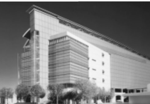
KONE is installing 20 TransVario™ escalators in Singapore's new Esplanade Mall shopping center.
