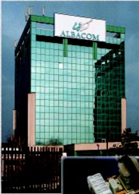
Helvar's SOLO dimmers and electronic ballasts were installed in the head quarters of Albacom, a telecommunication company in Milan, Italy.
