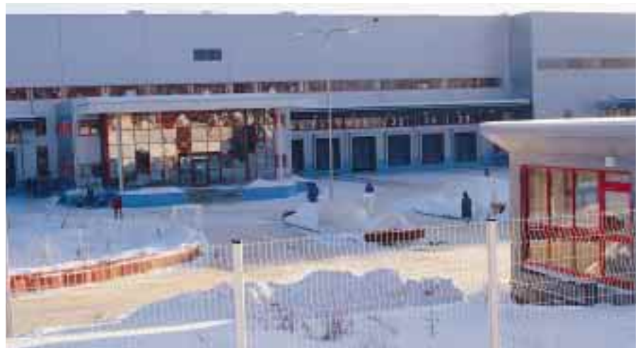
A logistics centre was constructed for a French client, Faure & Machet, near the Sheremetjevo Airport in Moscow.
