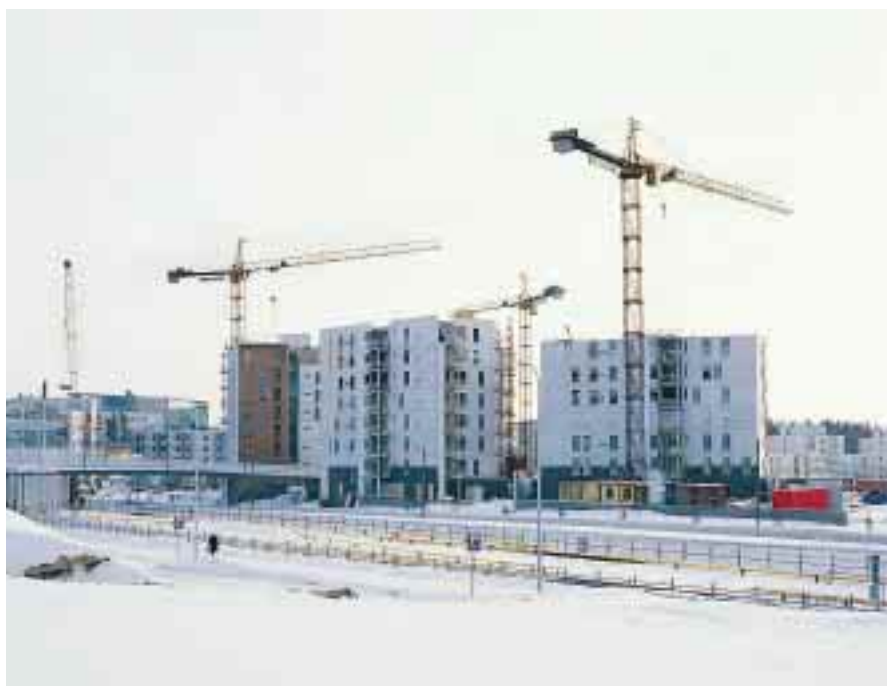
Three apartment blocks under construction in Helsinki.
