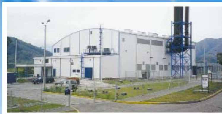
The 25 MW Pure Energy gas power plant supplied by Wärtsilä NSD to Cementos Diamante in Ibagué, Colombia.
