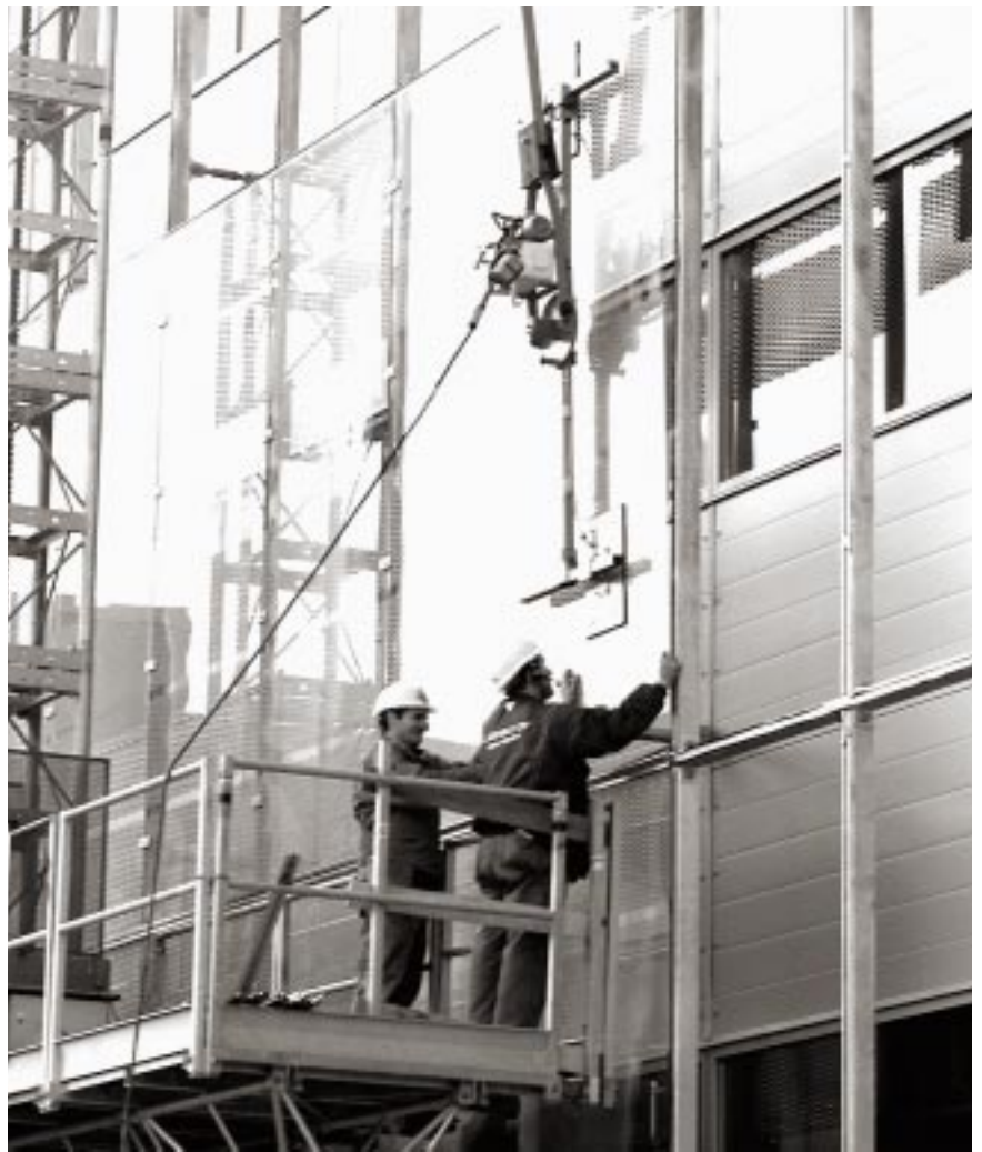
There was nothing to criticize at the Nokia building site.
