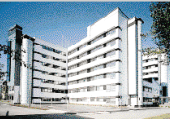
The Albatross Service Centre augments the new commercial centre in the Vuosaari district of Helsinki. The elegant façade is the first continuous glass surface of its size.
