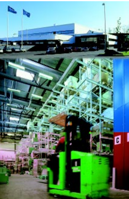
Office building of LVI-Dahl Oy, Vantaa.
