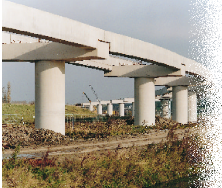
Short erection times and innovative solutions minimize traffic disturbances.
