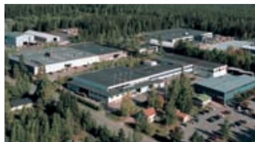
Hollola production plant
