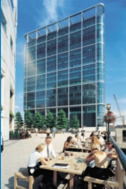
Citibank's new European Headquarters in the Canary Wharf section of London features 12 scenic KONE elevators.
