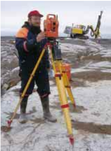
■ A new runway is being constructed at Helsinki-Vantaa Airport.
