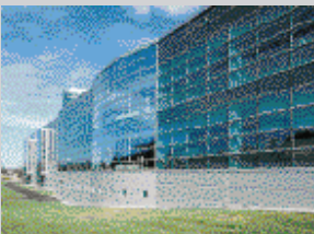
Tamglass Production Plant, Tampere
