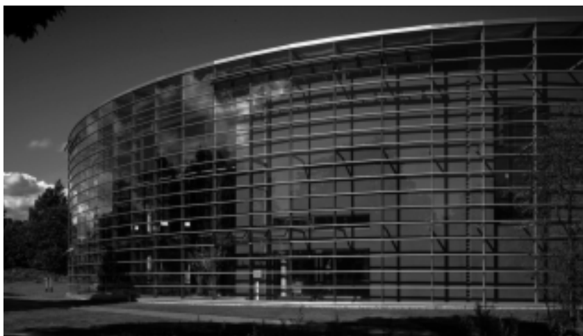
Nordic Aluminium's profiles on the facade of the Information Center of the Viikki scientific park in Helsinki.
