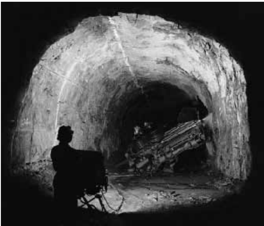
The use of remote-controlled machinery has improved working conditions in mining. Pictured is production face drilling in the Tara zinc mine in Ireland.
