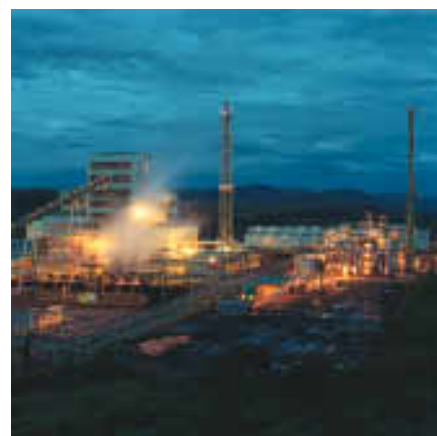
Outokumpu's core technology, the Flash Smelting Process, had its 50th anniversary in 1999. Direct Outokumpu Nickel Process, a new application of flash smelting without the separate converting, is successfully used at the Fortaleza Smelter in Brazil.
