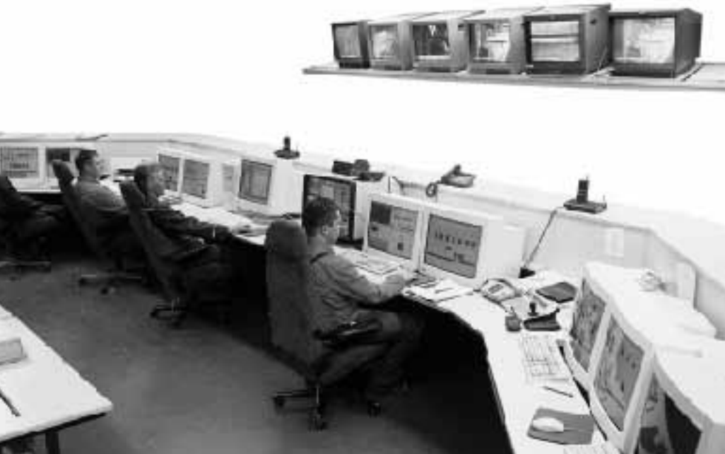
The Kokkola expansion project was completed at the end of 1998. During 1999 production ran at full capacity, 225 200 tonnes. Janne Marttila (left), Juhani Taivassalo and Veikko Erikkilä oversee the process in the new central control room.
