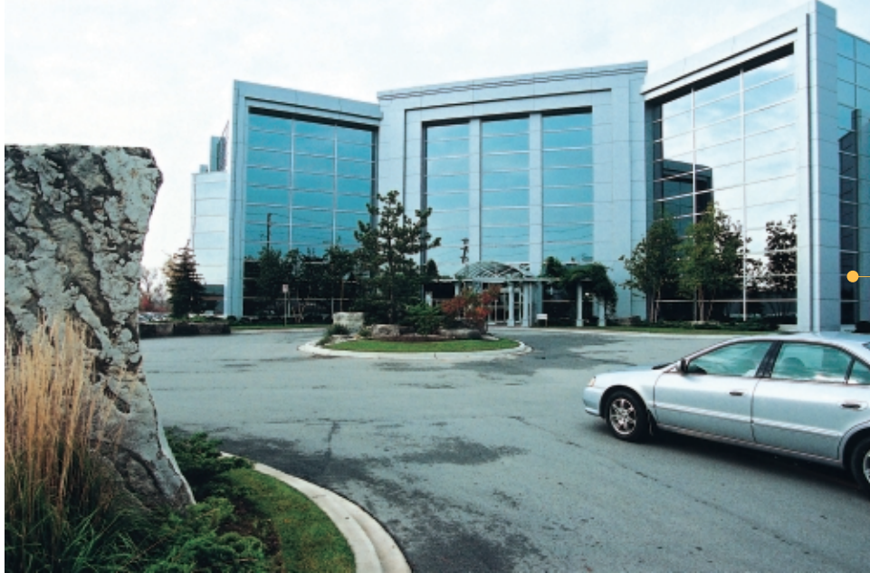
Raisio Chemicals also has skill centres in Canada, the UK and Korea. The centre in Canada operates on the ground floor of this building in Burlington, Ontario.
