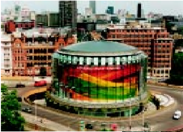
Gasell's Shine coated steel roofing was used in building this new cinema in London.
