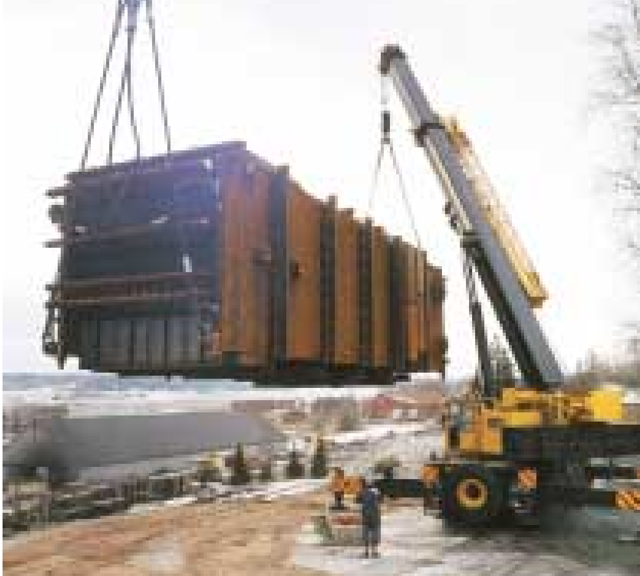
Voimavasu Oy, which was jointly established by Vapo Oy, Sucros Oy and ABB Service Oy, began construction of a 33 MW power plant in Salo in 1999. The plant's 85 tonne combustion chamber was installed in December.
