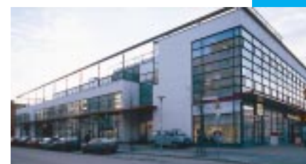
An extension to a metro station was completed in Ruoholahti.
