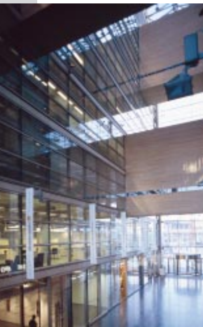
Sanomatalo Building, Helsinki: a heating and plumbing contract and a ventilation contract.
