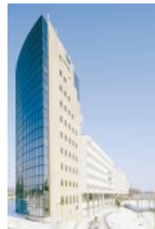
YIT Corporation's head office property is located next to the Käpylä Railway Station in Helsinki.
