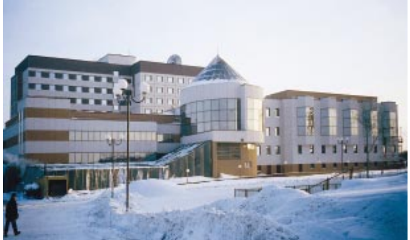
YIT performed the finishing works on baths of Kedrovij Log in Surgut, Russia.
