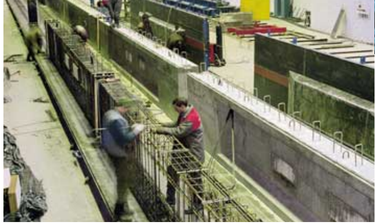
New production line for prestressed elements.
