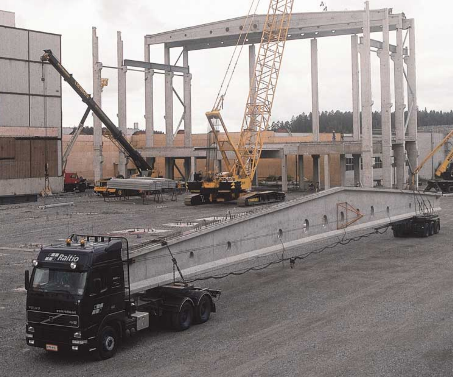
The demand for structural elements, like these 33.6 m long roof beams, grew during year 2000.
