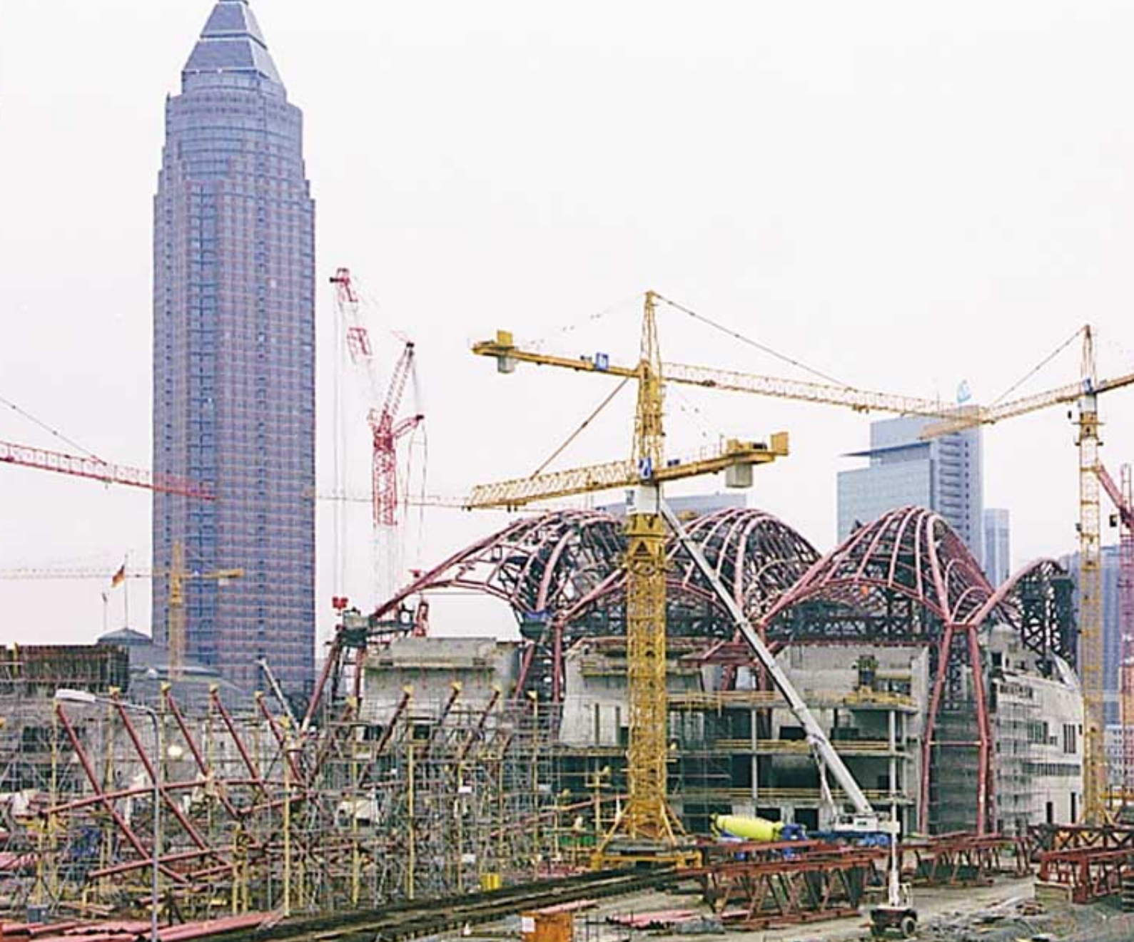
The combination of hollow-core slabs and steel structures is a popular alternative.
