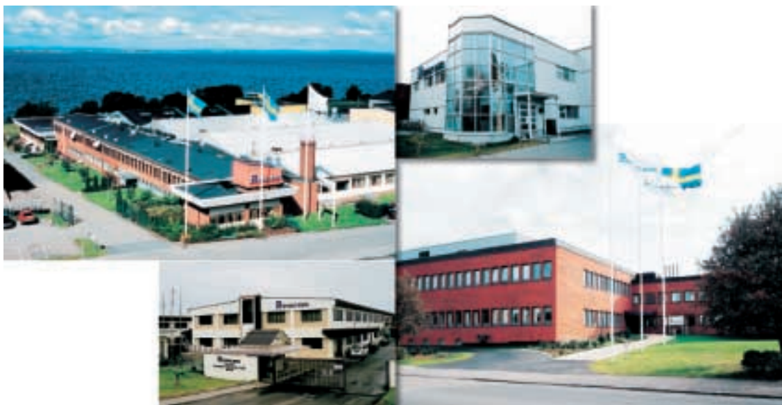
The modern manufacturing plants of Evox Rifa are located in Finland (Suomussalmi), Sweden (Gränna and Kalmar) and Indonesia (Batam). In 2002 manufacturing will be started in China (Nantong).
