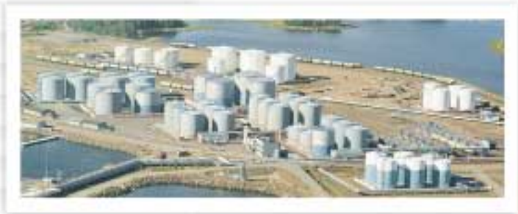
Transkem now has 30,000 m 3 additional storage capacity in Mussalo Deep Harbour in Kotka, Finland.
