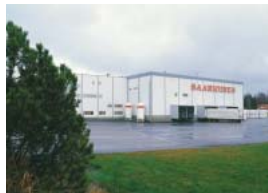
Thanks to the heat pump built by Sabroe Finland Oy, the Ruoka-Saarioinen food factory at Sahalahti is able to reduce its environmental load by a fourth.
