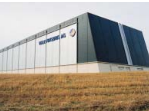
Altogether 13.000 m 2 of Prepan Danmark AS's own factory made PUR panels were used at Vejle Kole og Frysehus.
