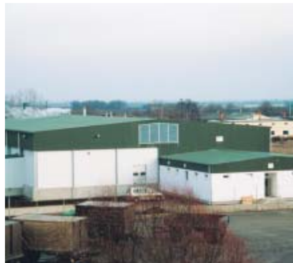
The biggest project Huurre Frigo Kft has ever undertaken, the Hungerit processing facility specializing in poultry products, was completed on 25 November, 2000.
