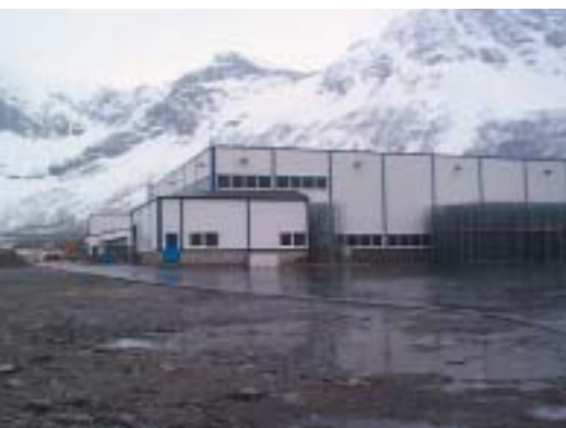
The construction area at the Klosterboer Terminal, Faroe Islands, built by Prepan Norge AS, totalled 3700 m 2 , of which 2600 m 2 are cold store facilities.
