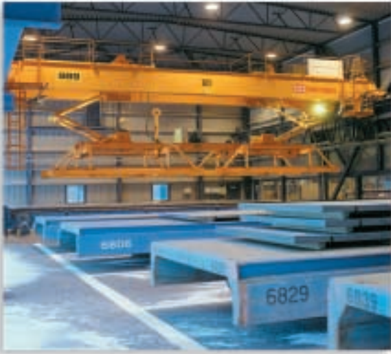
A fully automated overhead grab crane for lifting plate piles from the conveyor to carriers at SSAB's steel mill in Oxelösund, Sweden. The whole delivery included nine fully automated plate handling cranes.
