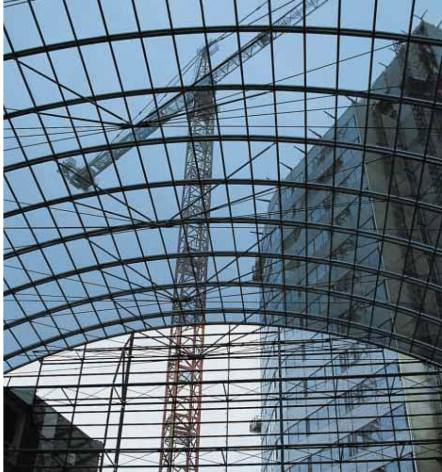
■ The electrical services and the telecommunications, security and data systems were installed in a new 17-storey office building on Itämerentori Square in Helsinki.
