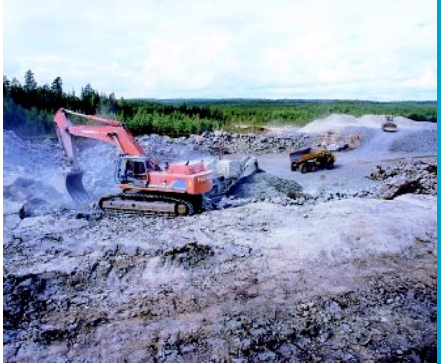
Natural gas trunk pipeline between Lappeenranta and Luumäki.
