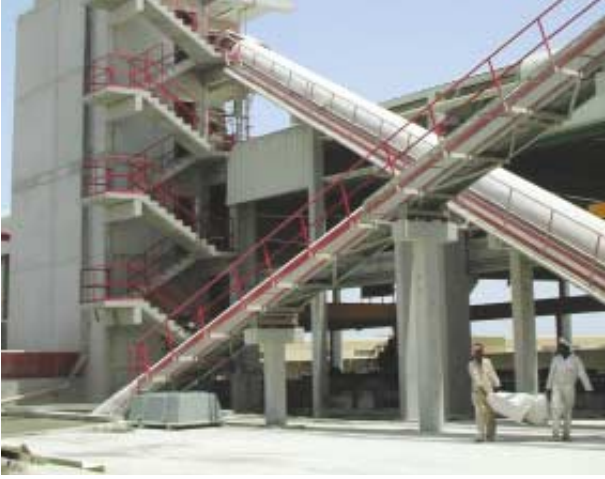
ELEMATIC Batching & Mixing plant lays a solid foundation for the manufacture of precast concrete also in Dubai.
