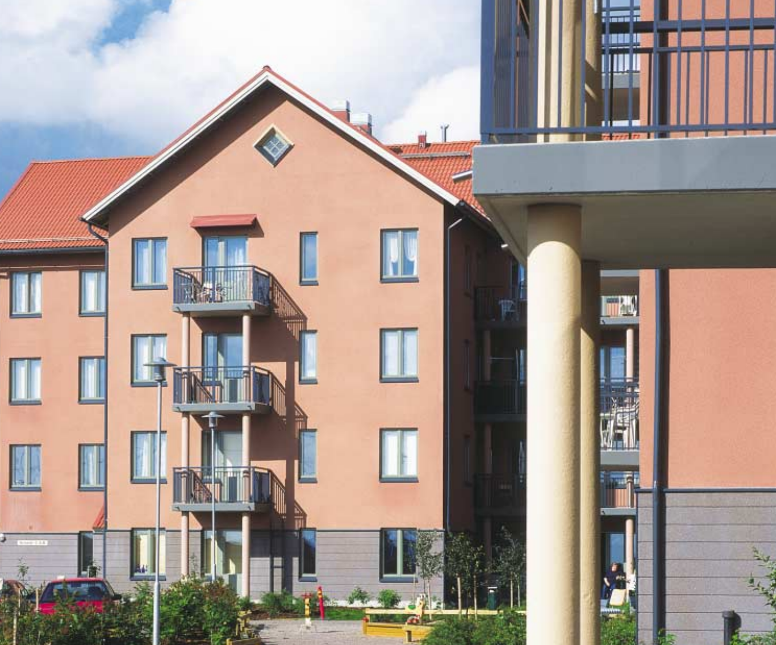
Apartment house with a jointless façade. The precast construction was developed in collaboration with the client.
