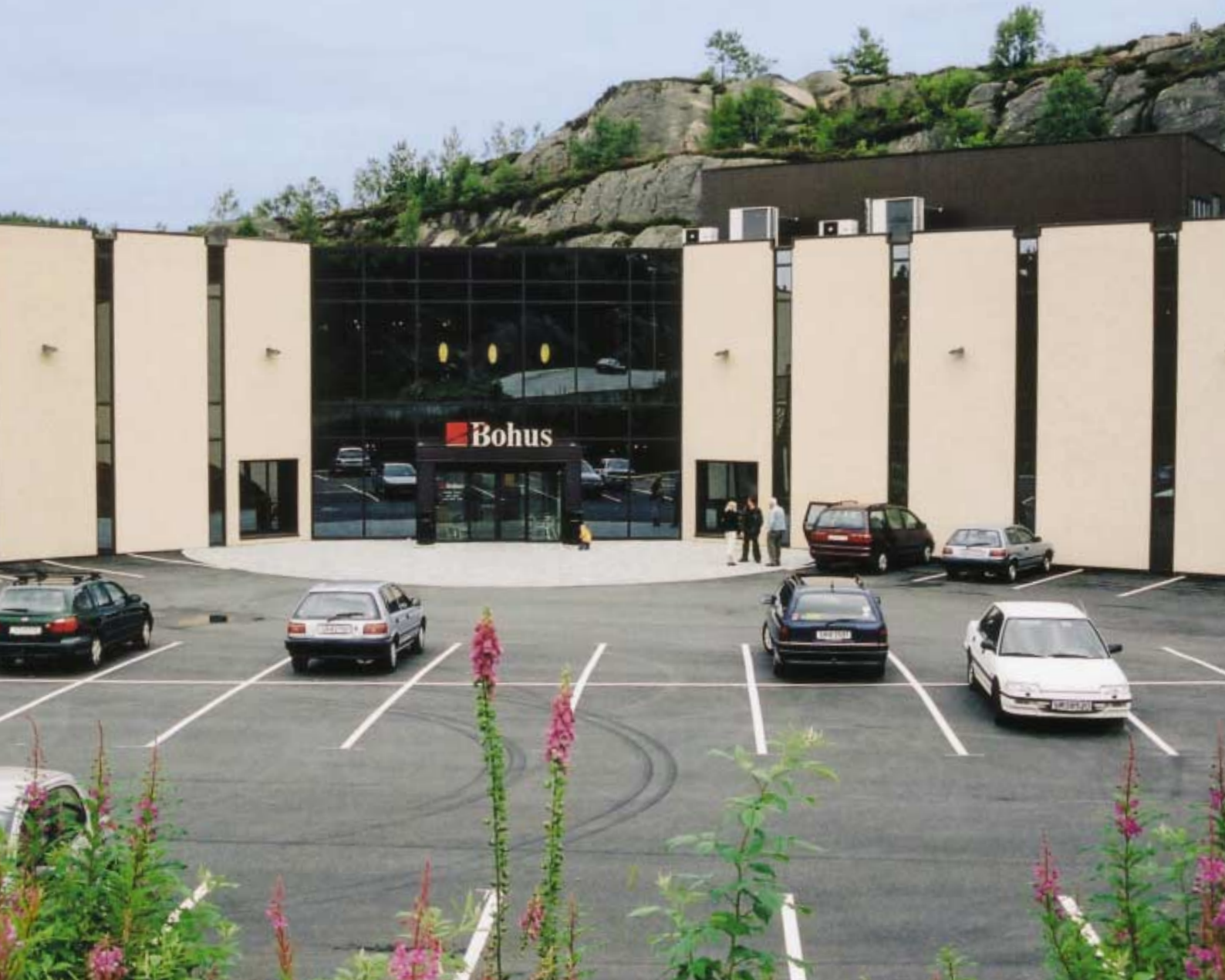
Bohus Drotningvik. Turn-key project – including precast façades, hollow core and roofing elements.
