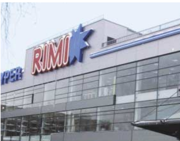
RIMI Hypermarket in Vilnius – the largest project in Betonika's history.
