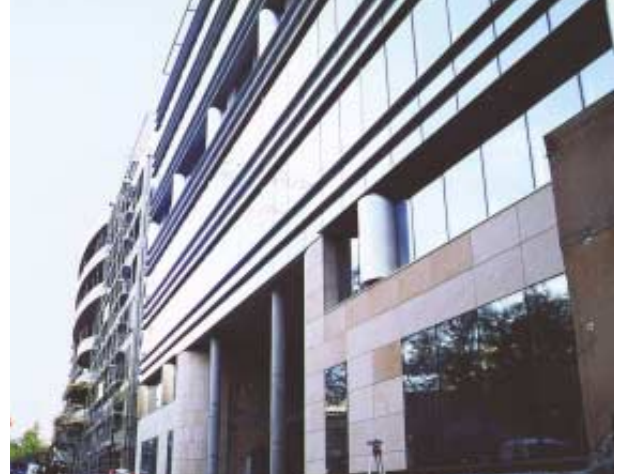
Frame elements formed an essential part of this office building in Warsaw.
