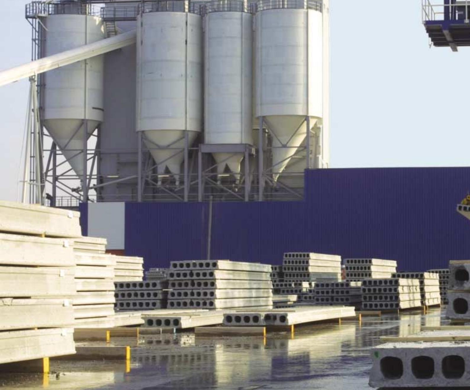
The new factory in Huissen with a hollow core slab capacity of 1 million sq metres was commissioned in the first half of 2001.
