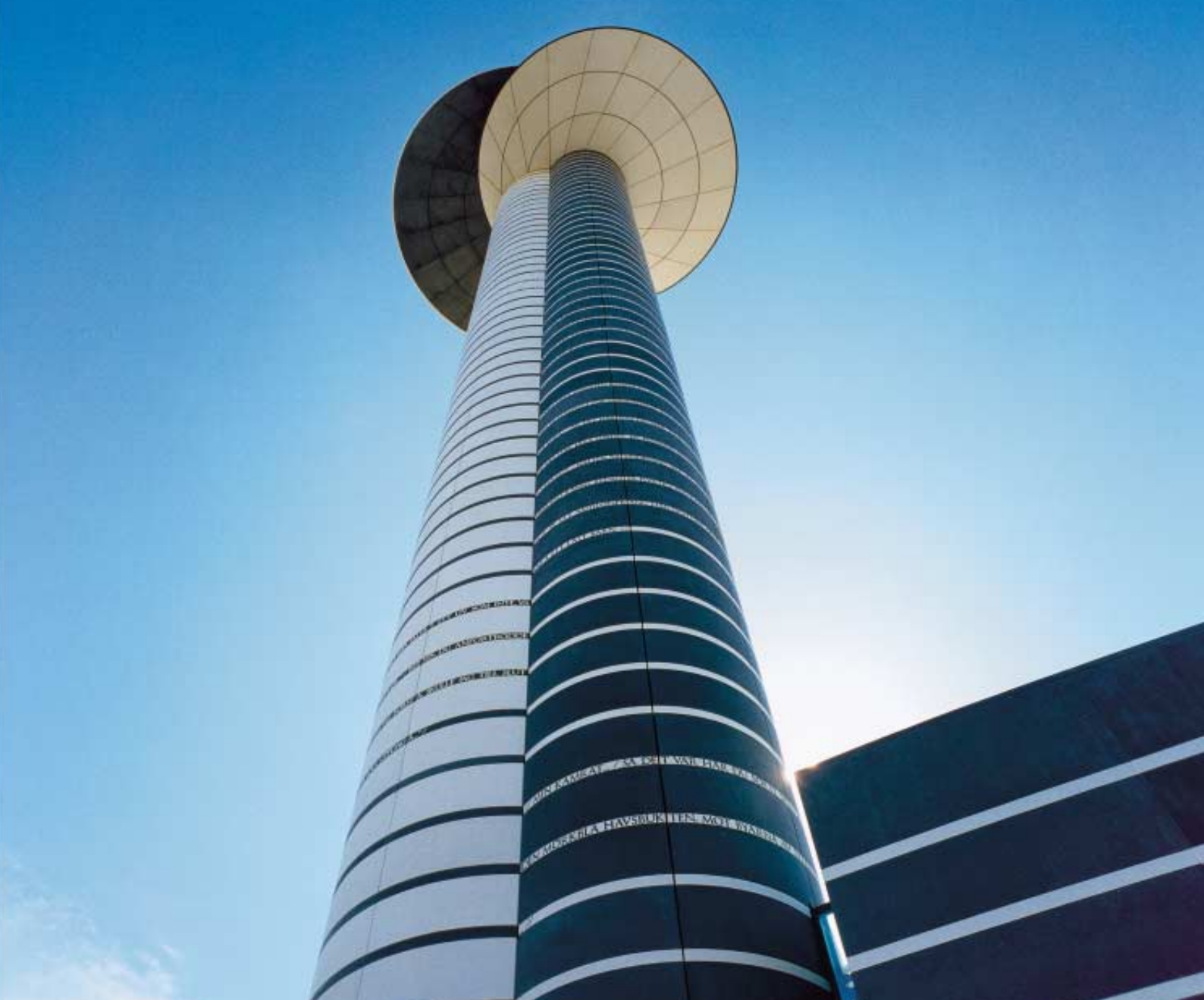
The new flight control tower at Arlanda Airport. The black and white cladding, manufactured by Strångbetong, is of polished concrete with intarsia letters.
