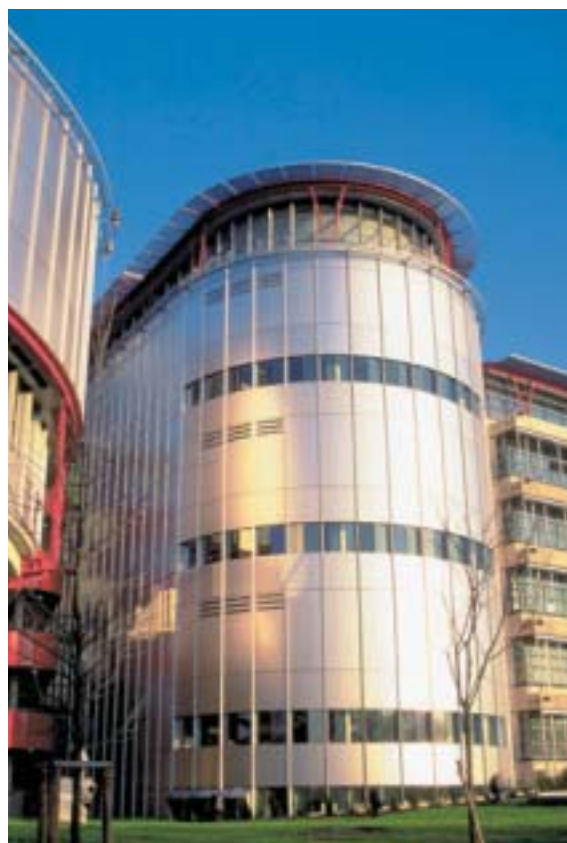
Stainless steel facade at the European Court of Human Rights in Strasbourg.
