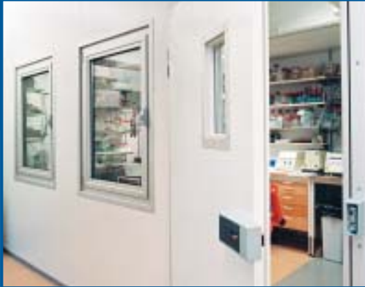
The refrigerated laboratory room in BioMedicinskt Centrum, Uppsala, Sweden, was delivered by Ki-Panel AB.
